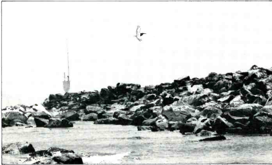
Marine beacon M, 310 kHz, Morro Bay, California. Operated and maintained by USCG. Power level 15 watts, signal has been copied as far away as the Oregon coast. (All photos this article by Michael Mideke)
